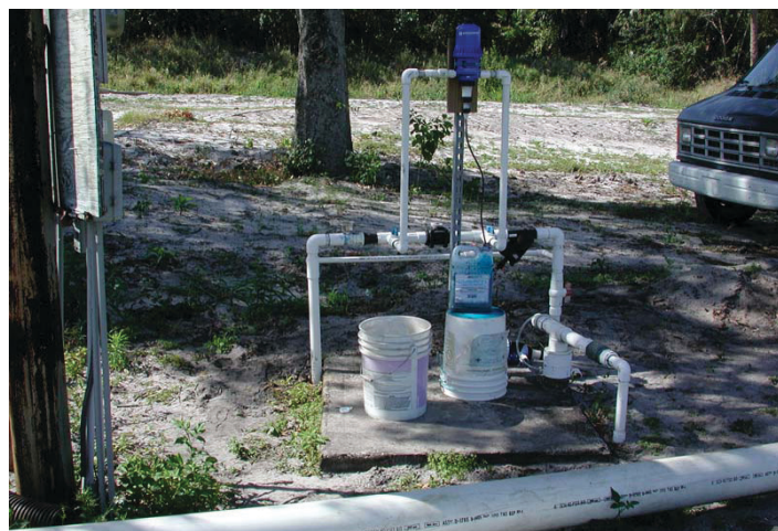
Figure 5. Injection made possible with a Dosatron. Credits: Eric Simonne.
